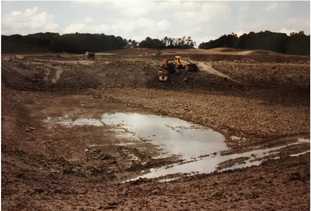
Photograph provided by client illustrating ground works and re-landscaping of 'West Park' to form the golf course in the 1990s. This is photograph illustrates the construction of the large lake.
