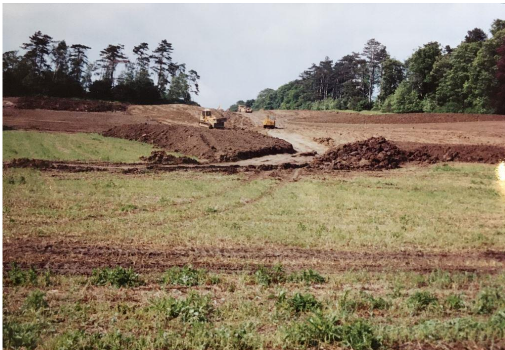
Figure 5: Photograph provided by client of ground works to form golf course in the 1990s. This shows the remodelling and cutting through of "Dalmeny Hill".
